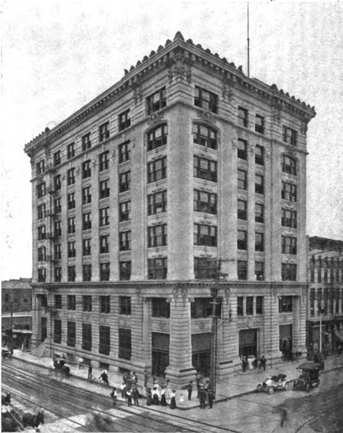
First National Bank Building, Houston, Texas
